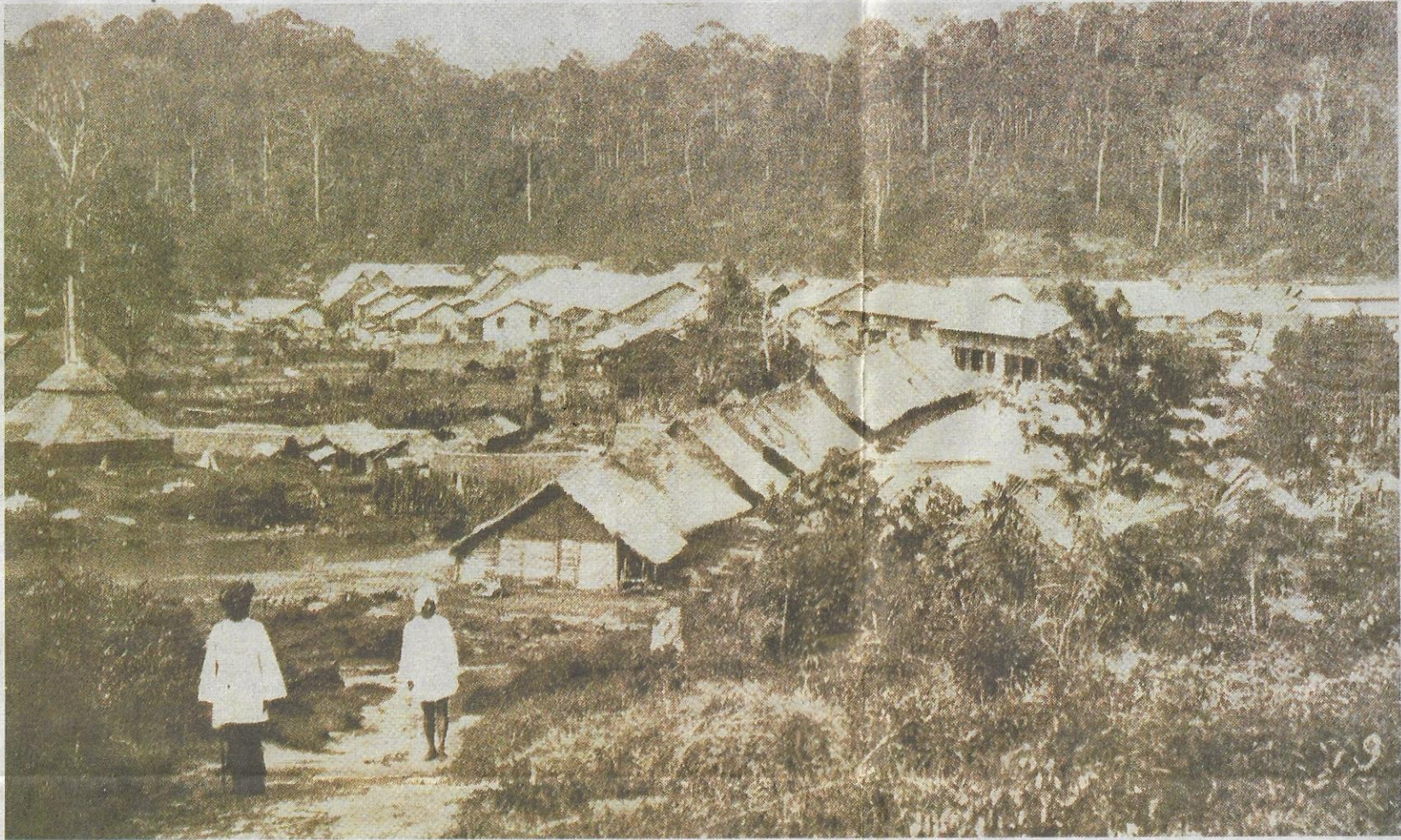
Kuala Lumpur in the 1800s saw the sprouting of wooden buildings to meet the needs of the growing population.
