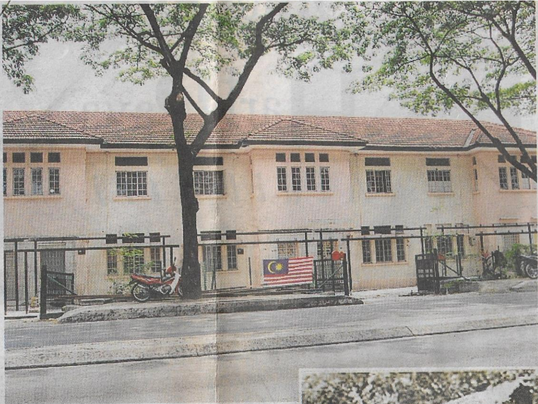
A facelift: Some of the quarters have been repaired and repainted.
