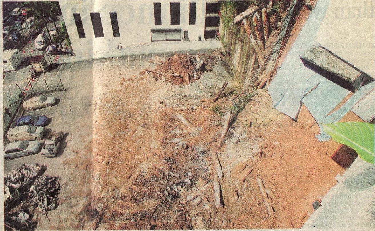
The landslide happened in the open-air car park between CIMB Commerce Square and CIMB Amanah building in Jalan Semantan yesterday. — NST picture by Mohd Radzi Bujang
