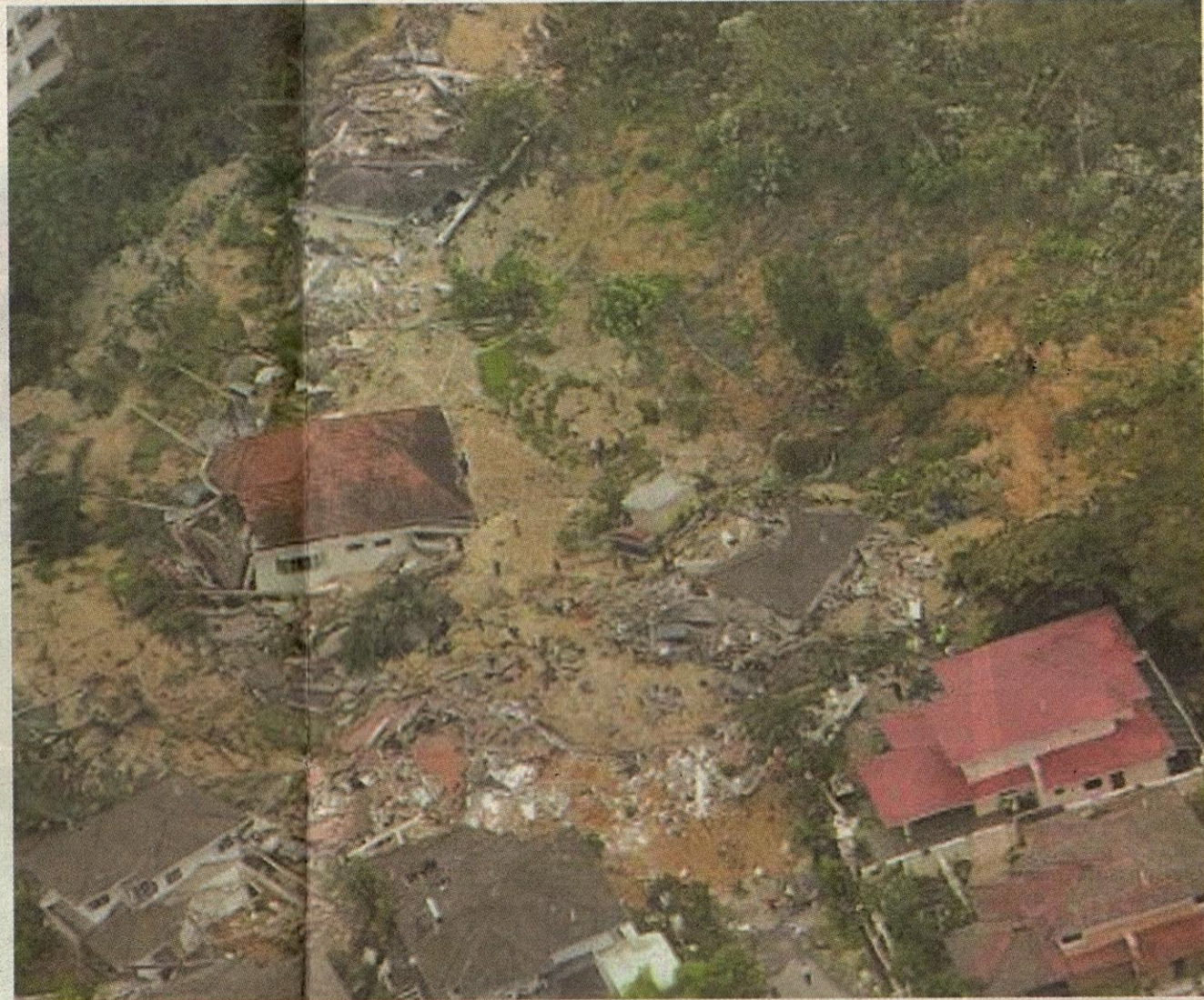
The Dec 6 landslide in Bukit Antarabangsa in Ampang, KL, killed four people, destroyed many homes, while over 3,000 residents had to be evacuated.
