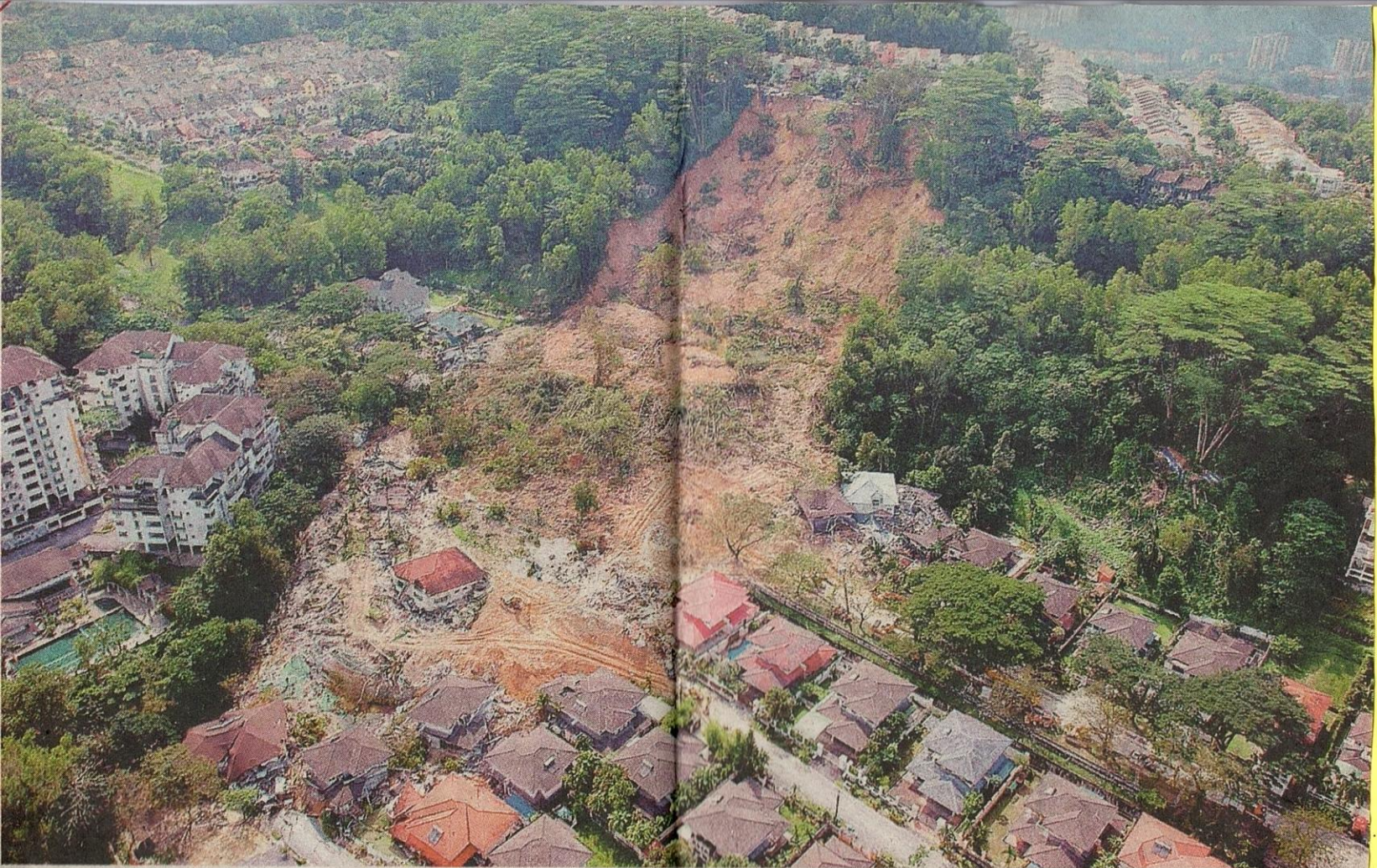
A file picture showing an aerial view of the Bukit Antarabangsa landslide that claimed five lives and flattened 14 bungalows on Dec 6 last year. Works Minister Datuk Seri Mohd Zin Mohamed yesterday announced a RM70 million budget to repair and reinforce the collapsed slope.
