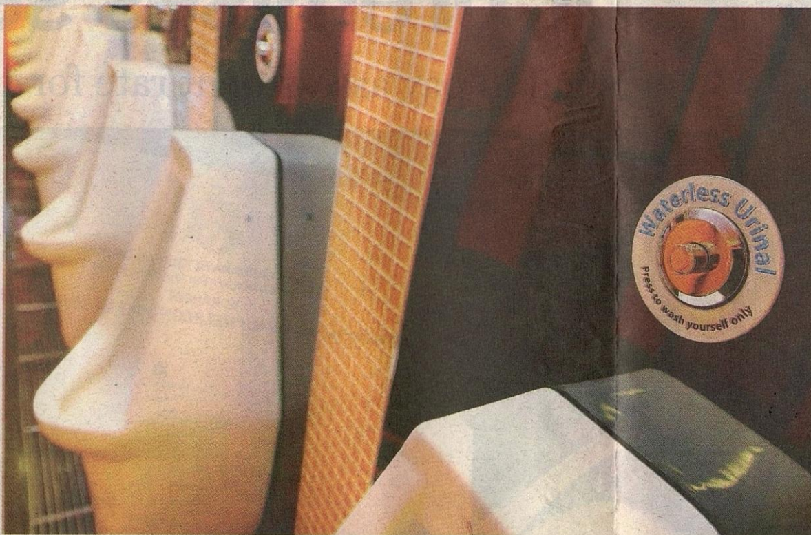
Waterless urinals: There is no need to flush at the urinals in men's washroom as each urinal is coated with BioCare Liquid, a special chemical that breaks down urine into environment-friendly components without using water.
