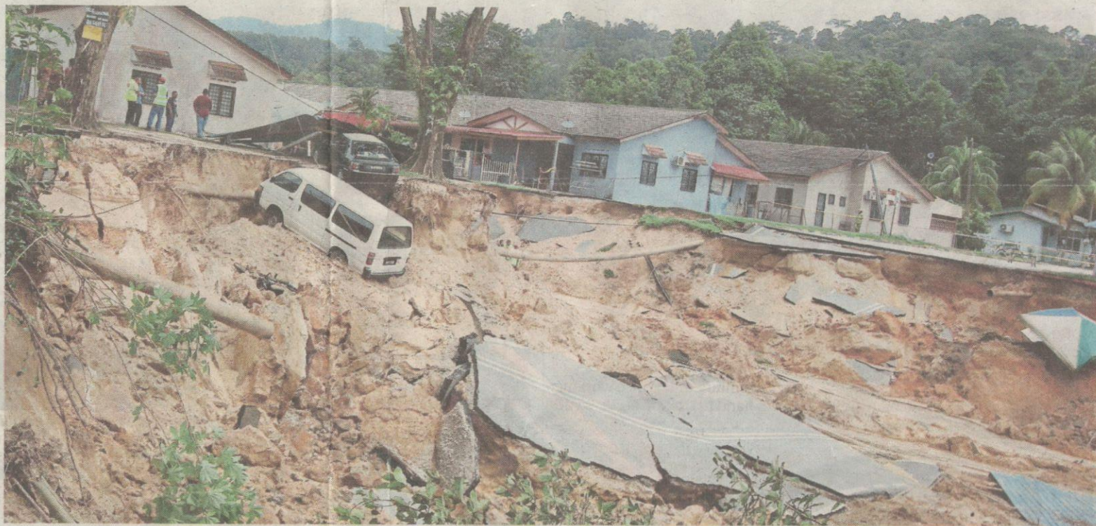
The sinkhole in Taman Idaman, Serendah, which was triggered by a landslide. Pic by Mohd Yusni Ariffin
