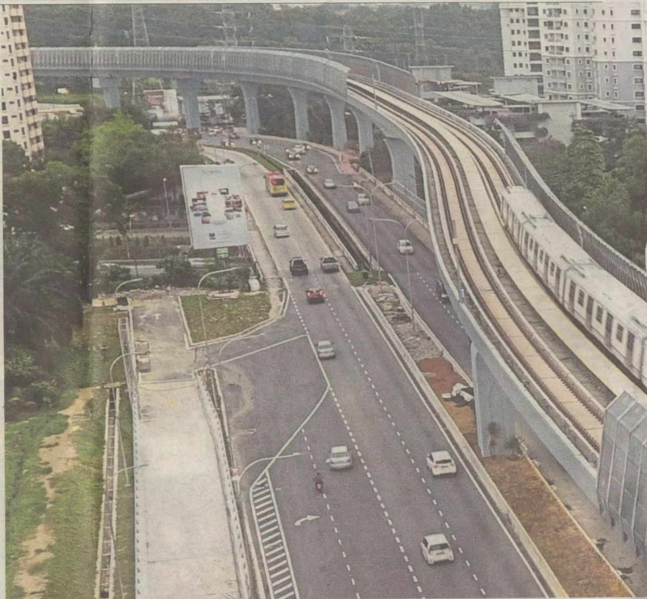
A test run of the MRT train at Sunway Damansara in Petaling Jaya yesterday. Pic by Zunnur Al Shafiq
