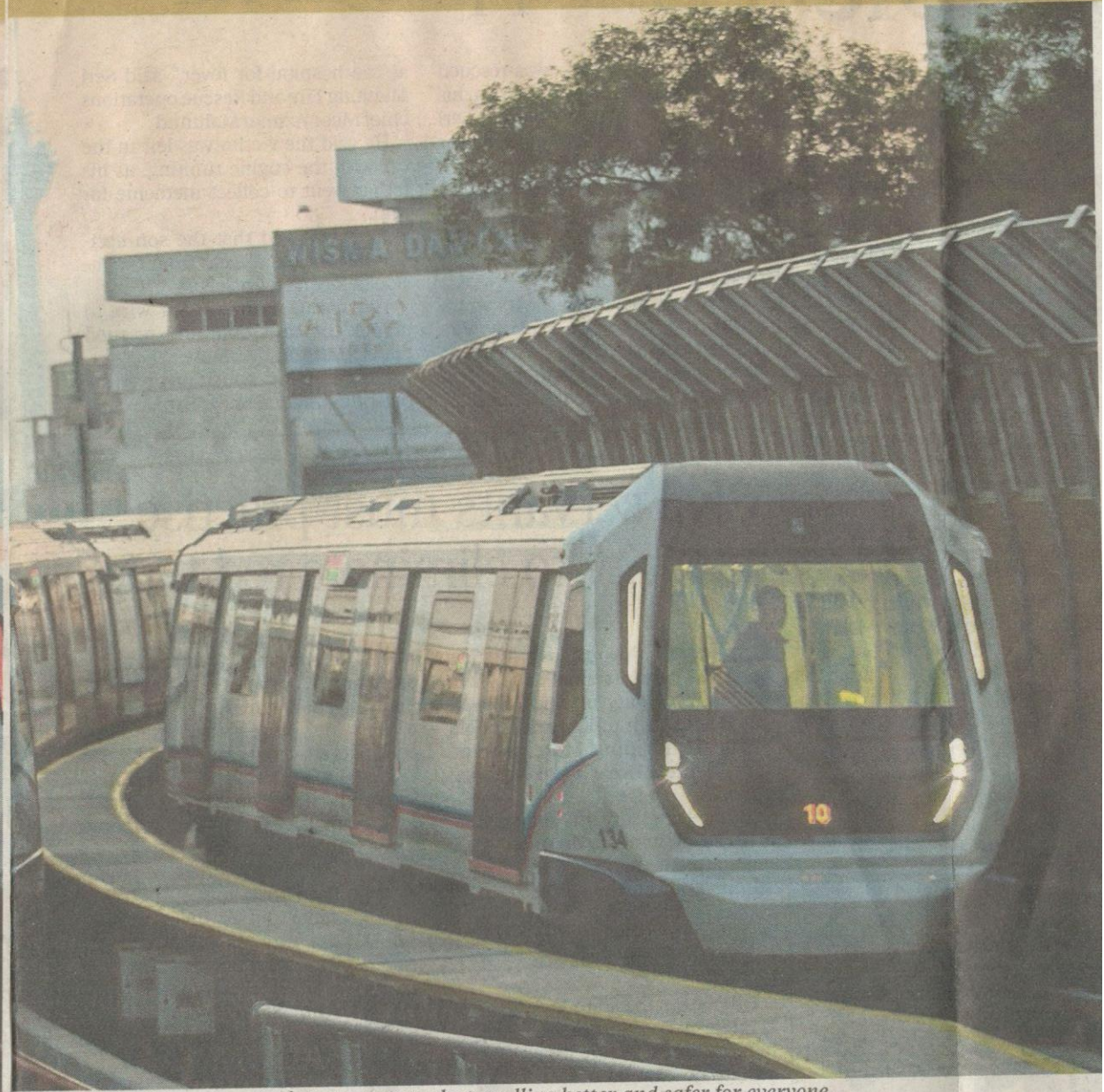
Efficient transportation systems make travelling better and safer for everyone.
